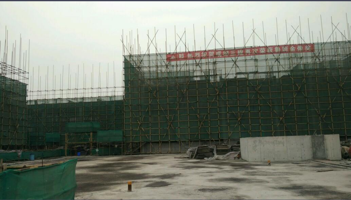
Chengdu Project R4 Site
